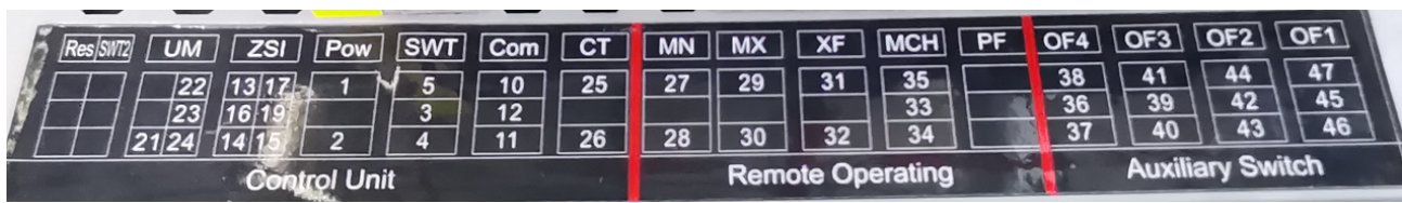
The terminal marking for control circuit
