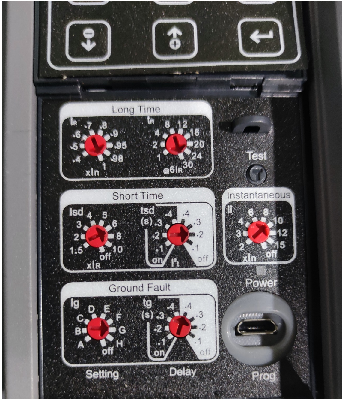
Dial switches for trip unit of type iTR326H and Genius 4.0H
